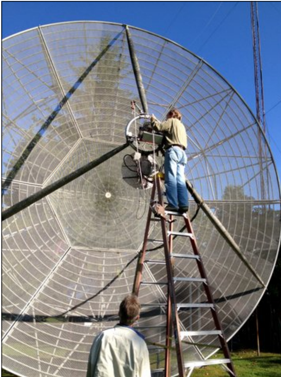
George, NE2U assists Al, K2UYH installing a microwave band feed on Al's "Kennedy Dish".
